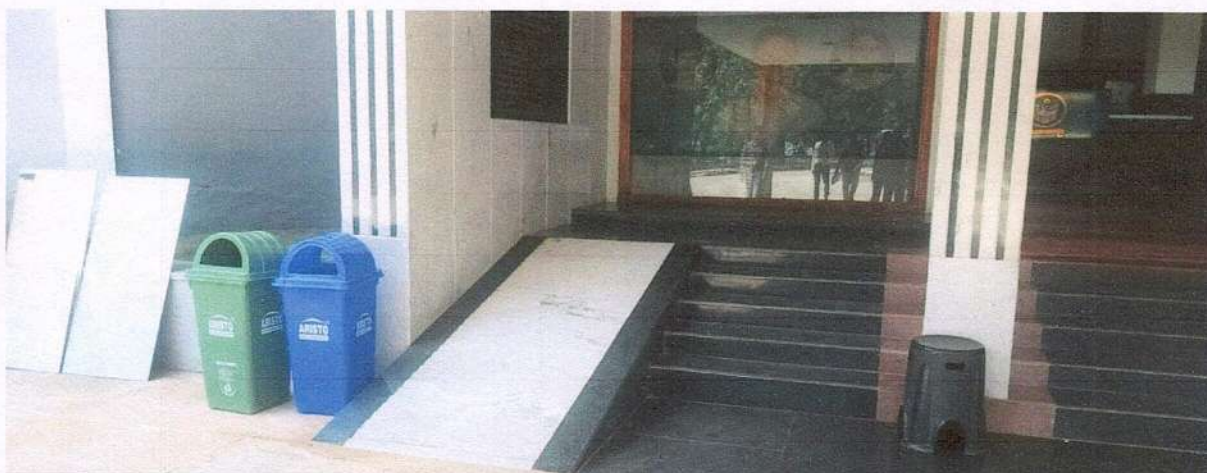
Ramp at Civil Engineering Block
