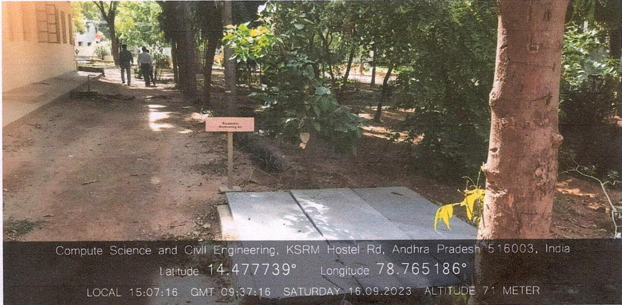
Rain Water Harvesting Pit near CE Block
