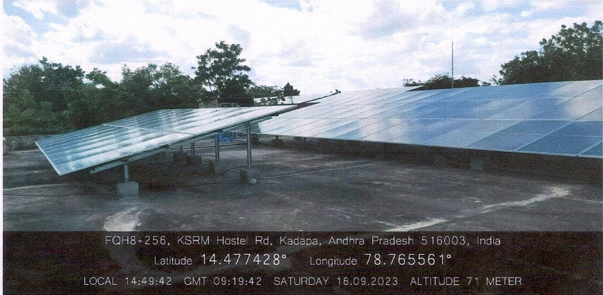
Solar Panels on the Rooftop of Civil Engineering Block
